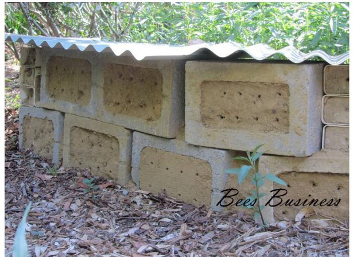
Rammed earth in Besser blocks, with roof for rain protection.
